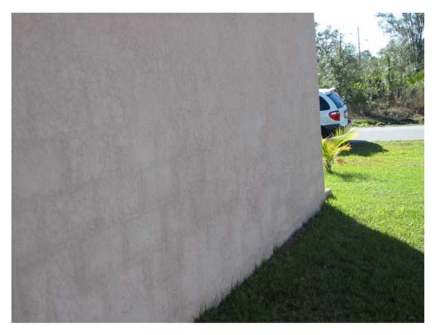
Factors affecting the ghosting phenomena include curing of the masonry wall, curing of the stucco and thickness of the plaster.
